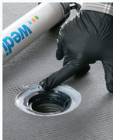
Attach the drain flange. Joint sealant goes below the flange, and a threaded collar pulls it tight. More sealant goes over the top.
