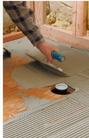
Apply thinset. Apply a notched coat of thinset mortar to the back of the pan and the subfloor.
