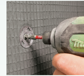
Specialized fasteners. Wedi's screw and washer system attaches the panels securely. Drive them carefully, just flush with the surface.
