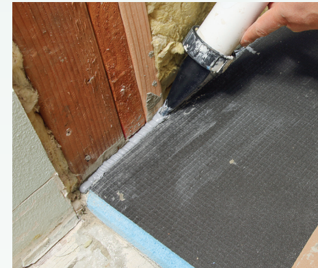
Apply sealant. The pan is rabbeted to accept the wall panels. Apply a full bead of sealant along each notch.
