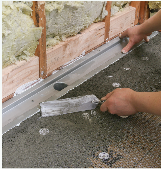
Custom drain. I'm using a Laticrete linear drain here, setting it in the dry-pack mud-bed shower pan before installing the bottom piece of foamboard over its back edge.
