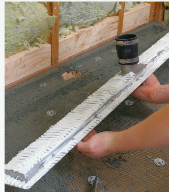
Custom drain. I'm using a Laticrete linear drain here, setting it in the dry-pack mud-bed shower pan before installing the bottom piece of foamboard over its back edge.
